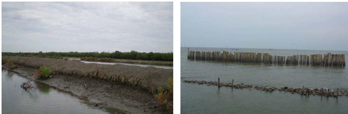
Figure 5.3 Heightening of dikes (left) and a concrete-pole breakwater (right)
