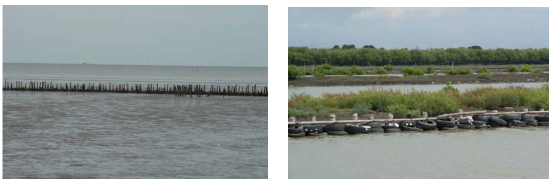
Figure 5.6 Part of the BMA-constructed stone breakwater (left) and a tire breakwater (right)
