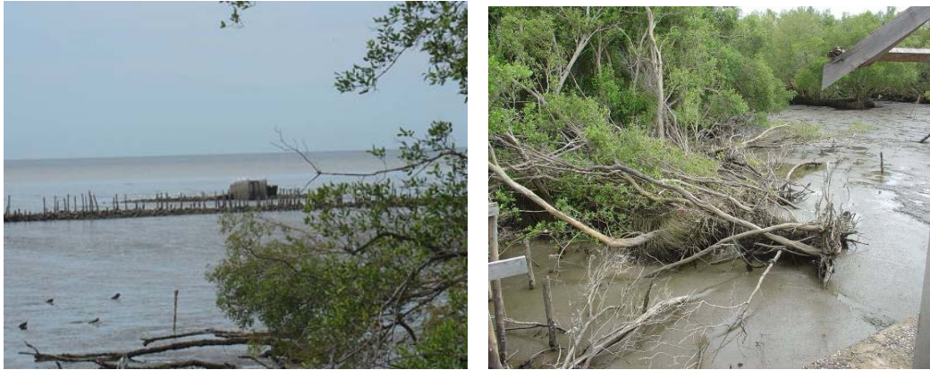
Figure 3.3: An old pond's gate that is no longer used (left). Mangroves felled by strong waves (right).
